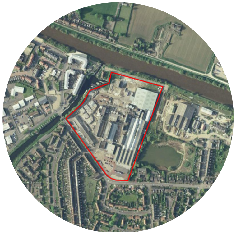
Google Earth image from 2007 showing the former Paper Mill buildings on the site.
