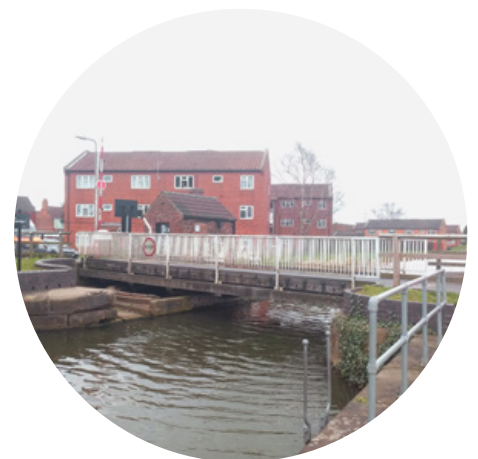
From left: Lock keeper's cottages; Lock bridge; Swing bridge Denison Rd
